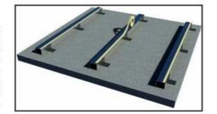
b. Apply the 896 PanelFix adhesive to the substructure and directly onto the panel. The adhesive should be applied continuously with a caulking gun (minimum 5mm from the tape). Extrude a wide bead of silicone to achieve the required joint dimension. Remove the protective layer from the tape after the adhesive application.
